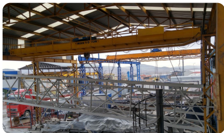
Workshop with 10 t overhead crane
